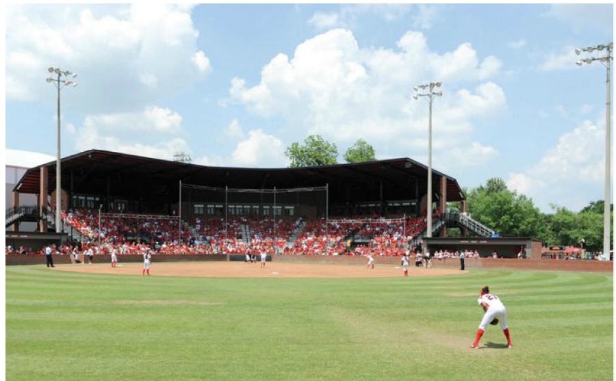
Louisville Softball Field
